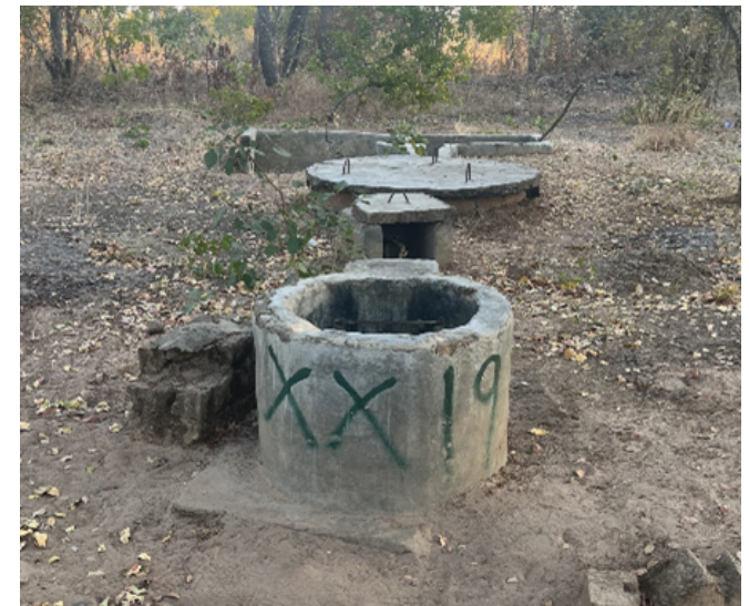
Above: onsite biogas digester
